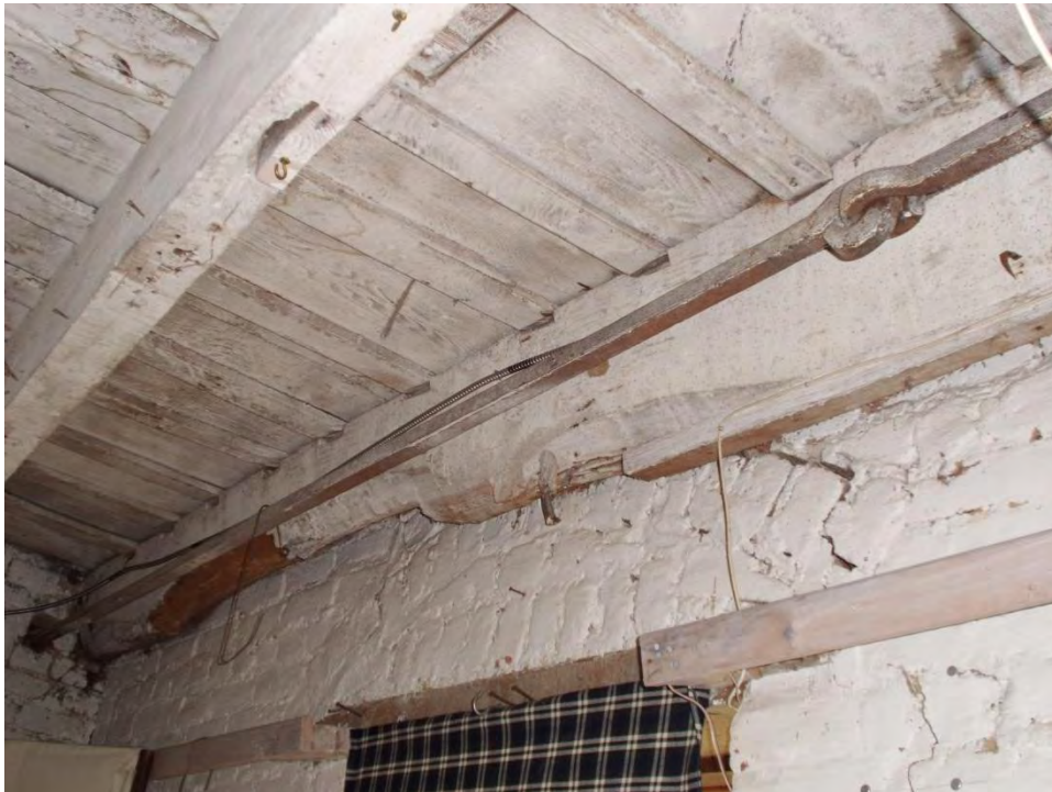
Figure 22: Tie rod at west gable wall
