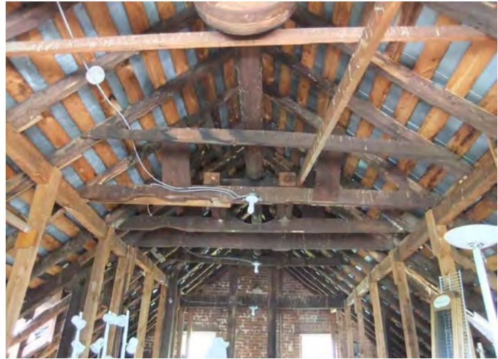
Above: Roof framing with rafters, collars and purlins on stud posts.
