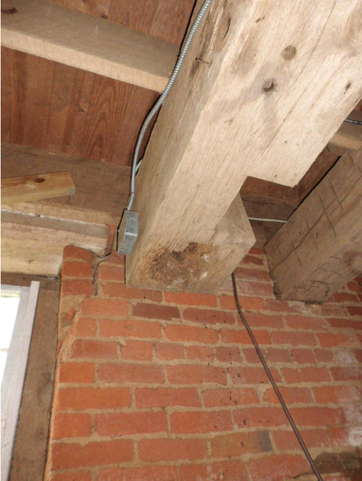
Figure 43: Hurst frame beam with loss of supporting post and cracked masonry at opening to left
