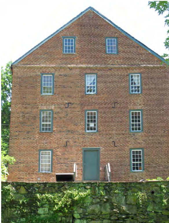
West End, Waterford Mill, 2012. A double row of projecting bricks can be seen above the third-floor windows.
