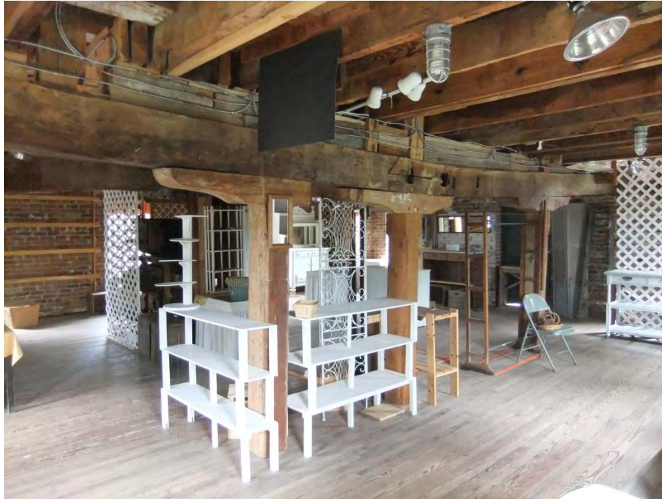
Figure 19: Third floor relocated column and beam deflection
