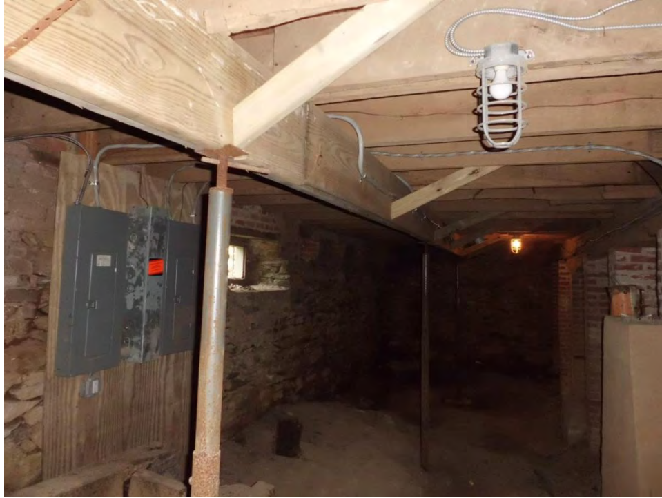
Figure 35: First floor shoring within northern joist bay
