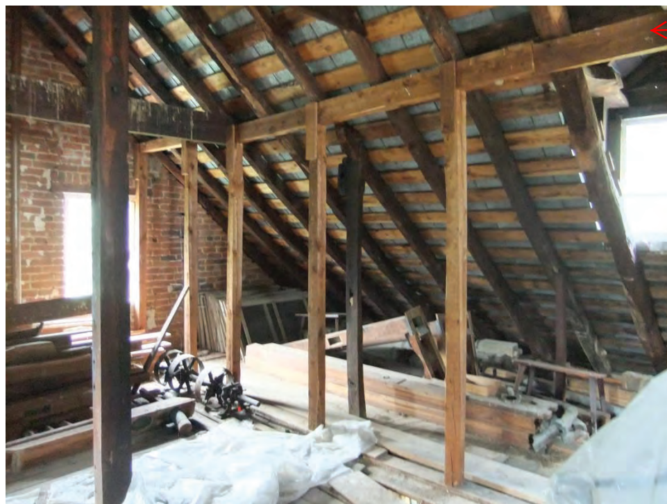
Figure 6: Roof purlin and post support
