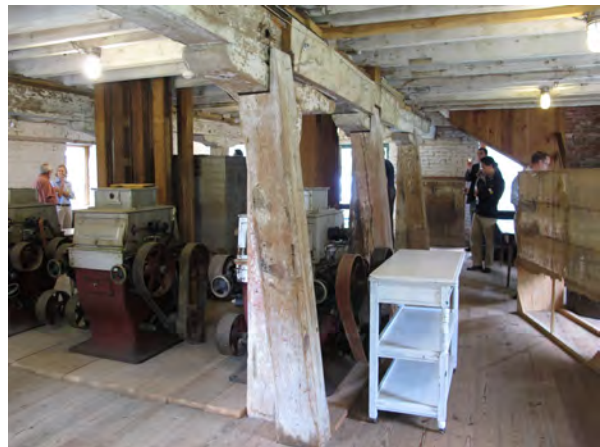
First floor looking east from south structural bay showing added braces and roller stands.
