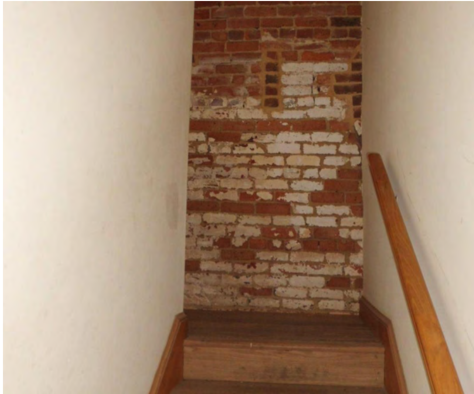
Figure 31: Brick spalling within northwest stairwell landing
