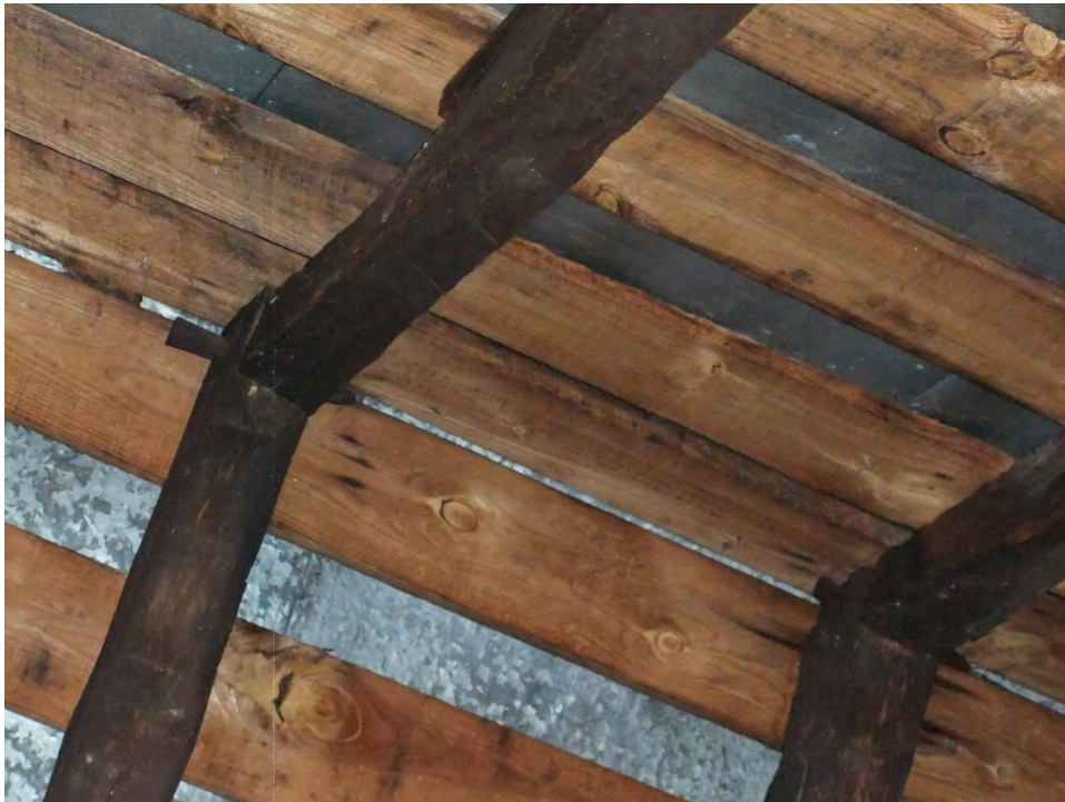
Figure 4: Roof rafter pin connection at ridge
