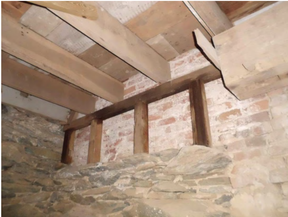
Figure 38: First floor southern joist wood knee wall
