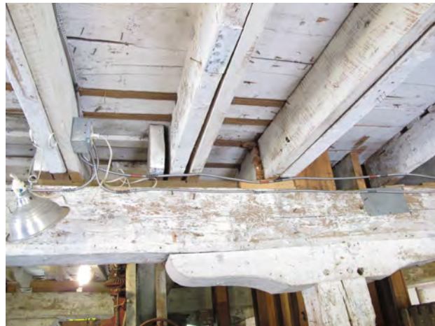
The southeast post on the first floor, showing typical blocking and sistering performed in 1983-4.
