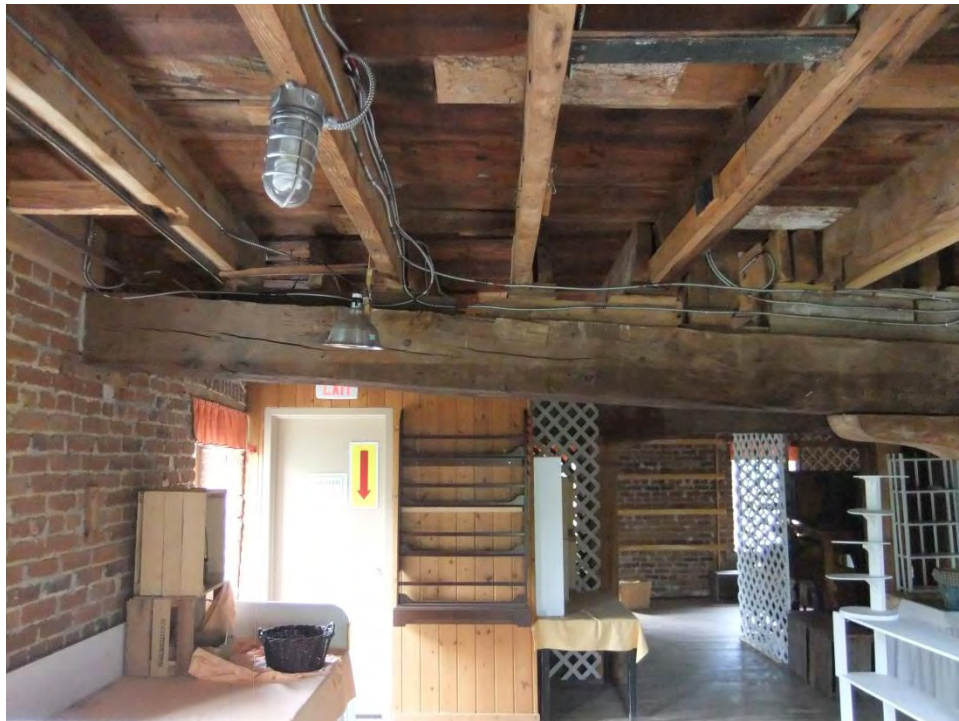
Figure 18: Third floor beam deflection
