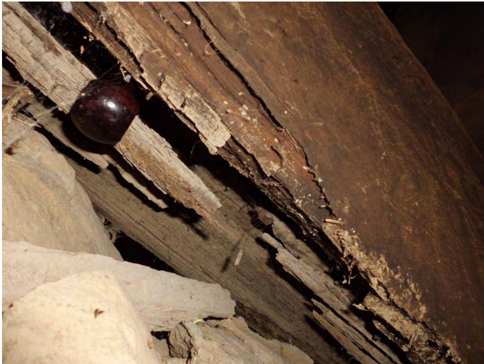
Figure 45: Hurst frame deterioration
