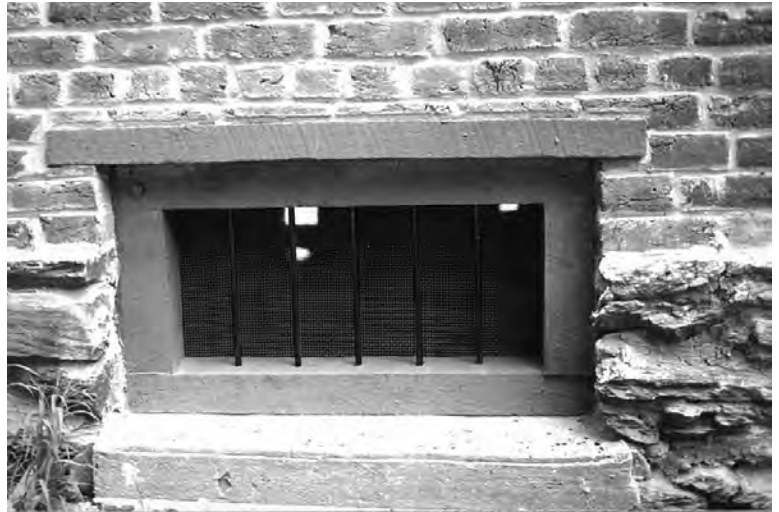
New basement vent in center of north wall.
