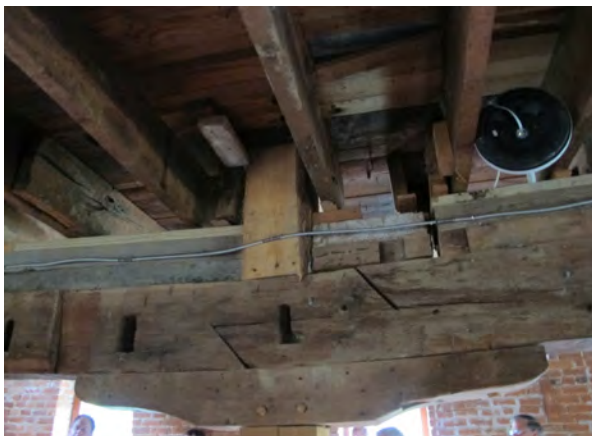
Typical scarf joint, center of northern beam on second floor.
