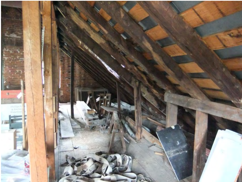
Figure 8: Intermediate support of rafters
