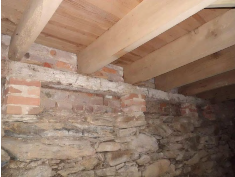
Figure 37: First floor northern joist masonry pier support
