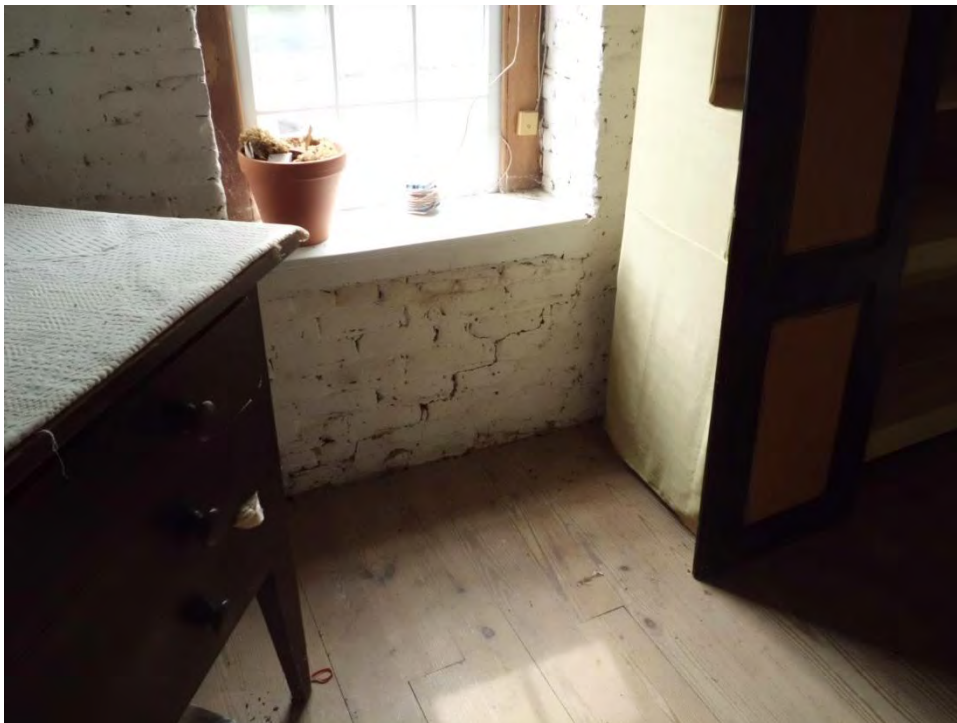
Figure 30: Diagonal cracking within mortar joints below first floor window opening along west wall
