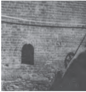
Westernmost of the upper arches in the south wall in the 1930s (above left) and today (above right). It and the brickwork around have not been greatly changed. The crude rowlock arch does appear to have been inserted in the later 19th century- note the neat section of running bond to the right of the opening that does not match the rest of the brickwork.
