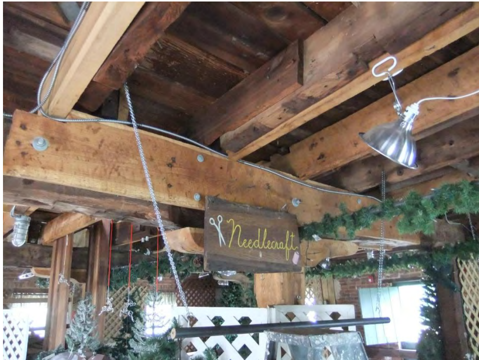
Figure 10: Attic level longitudinal beam sister reinforcement
