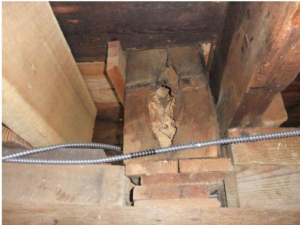
Figure 20: Third floor post deterioration
