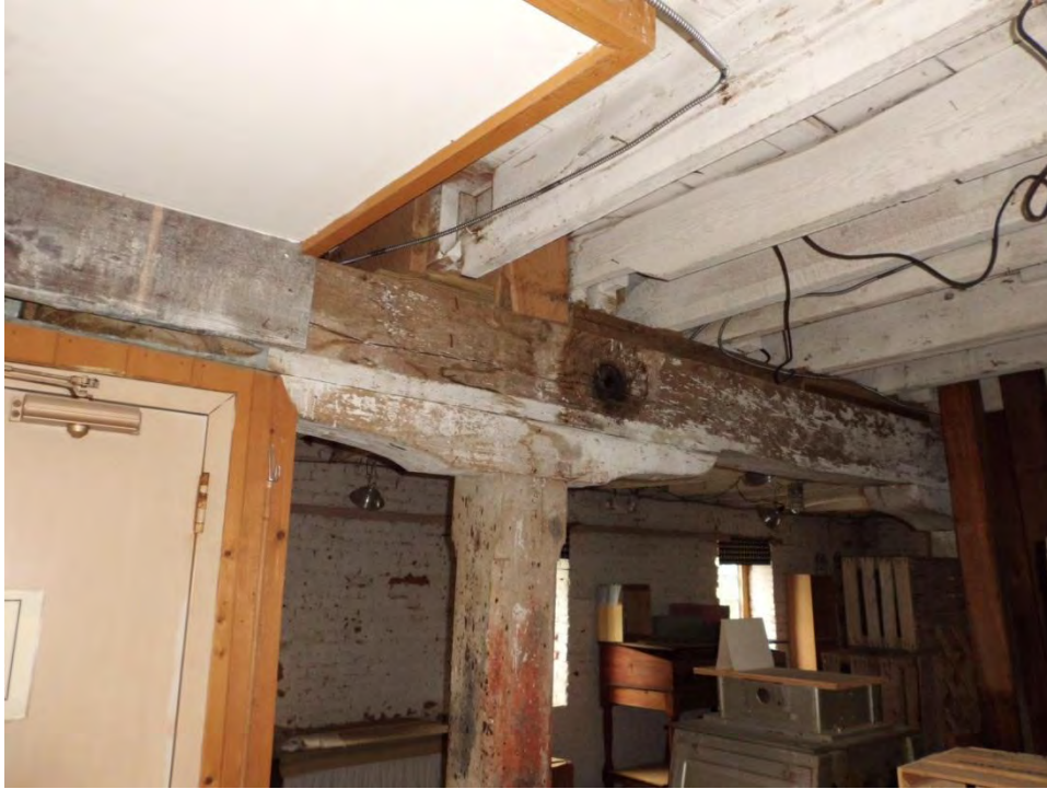
Figure 25: Second floor longitudinal beam notch
