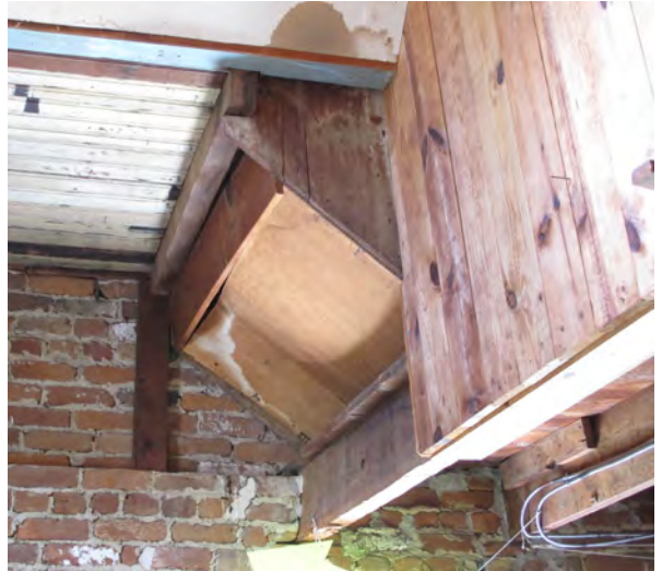
The upper flight of the stair from the second to the third floor, showing nineteenth-century stringers.
