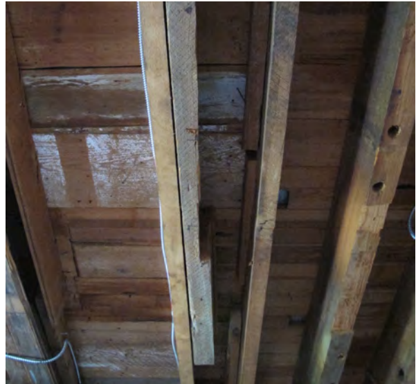
Above: The two sets of peg holes on the right (located near the west end of the center structural bay) are probably the location of a support for a central longitudinal second-floor power shaft. Looking north at Joist 18, Zone B, Sheet A-15 on the 1983 record drawings. The floor to the left is mostly old and to the right is replaced.
