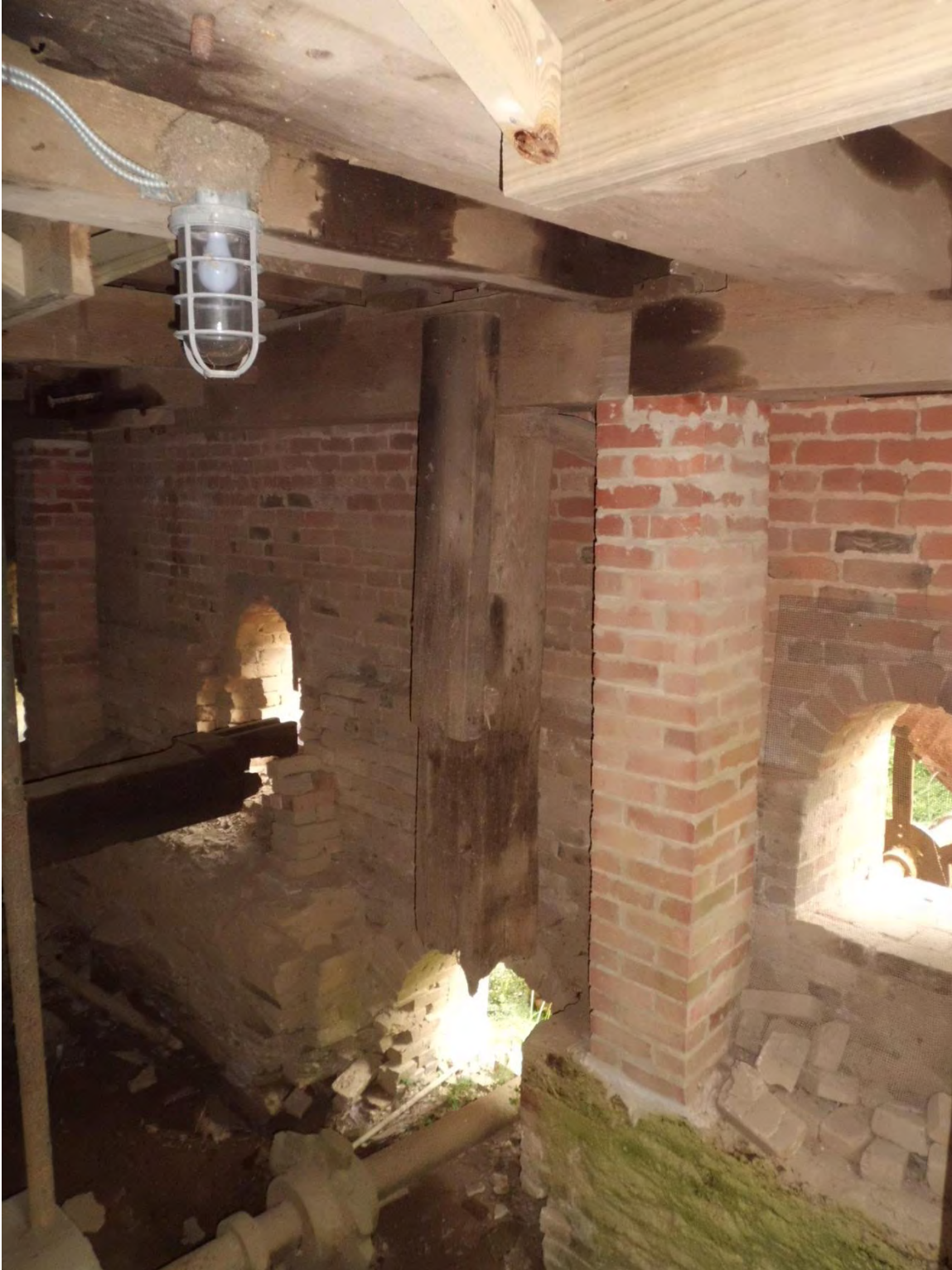
Figure 39: First floor joist supported on Hurst frame
