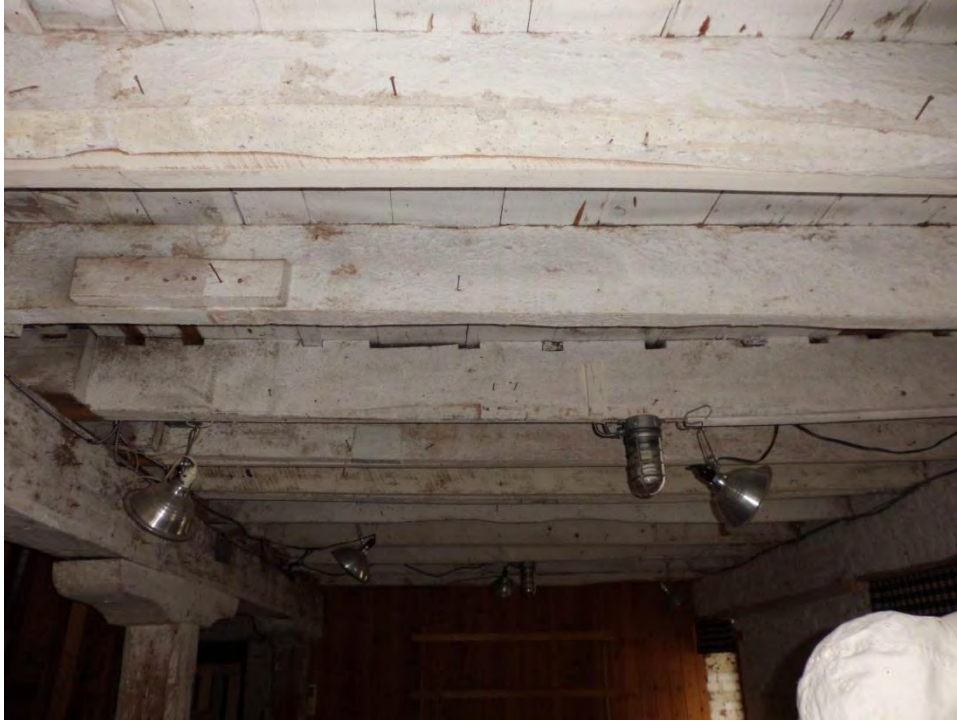
Figure 21: Second floor joist framing
