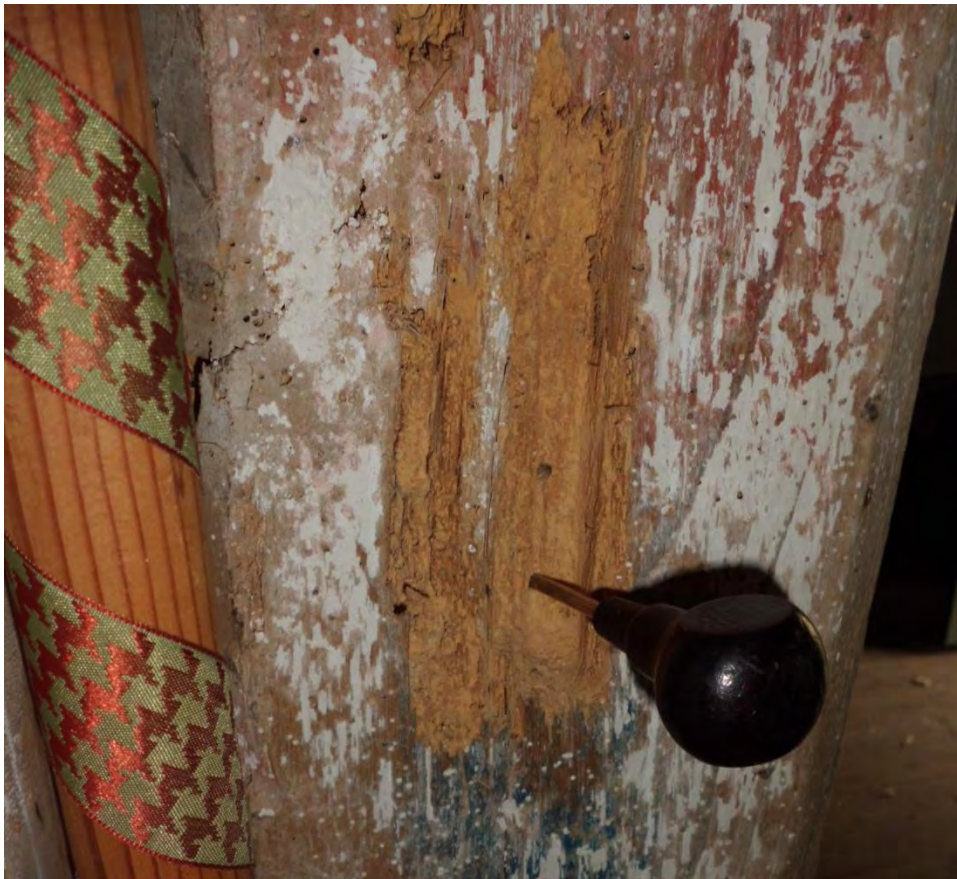
Figure 26: Second floor southeast corner column deterioration
