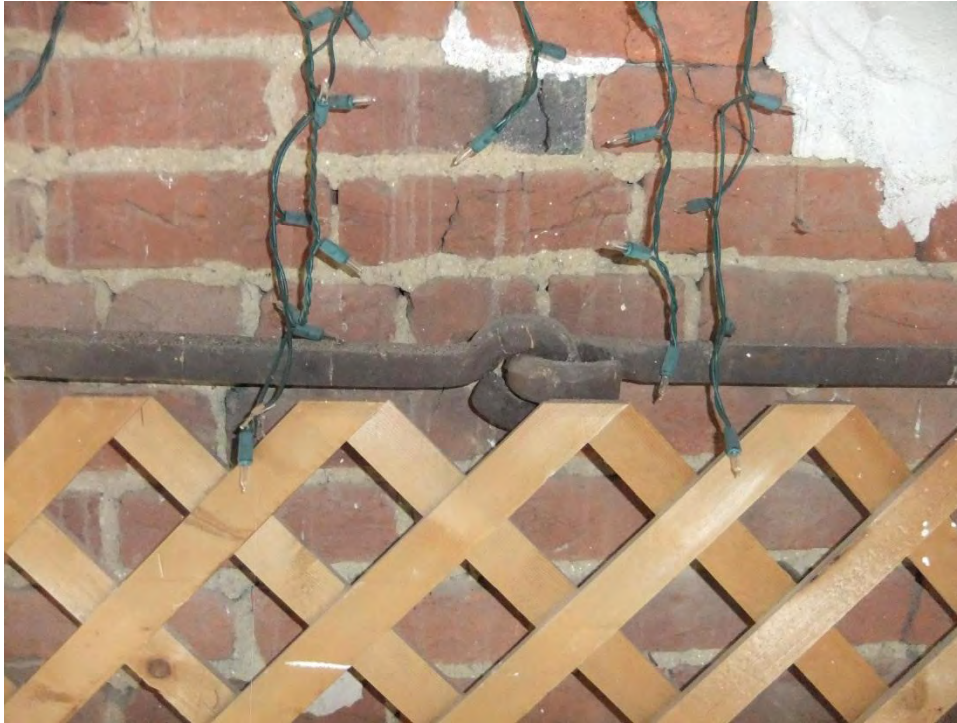
Figure 13: Attic level square tie rod connection
