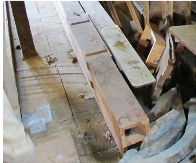
Right: Traces of a hopper boy flight arm on the attic floor
