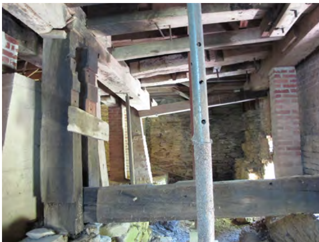
The hurst frame looking east with the surviving bridge beam in foreground.
