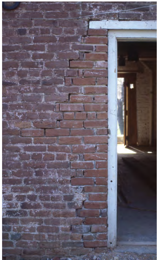
East entry door brick during repair, April 1984 [WF slide collection]
