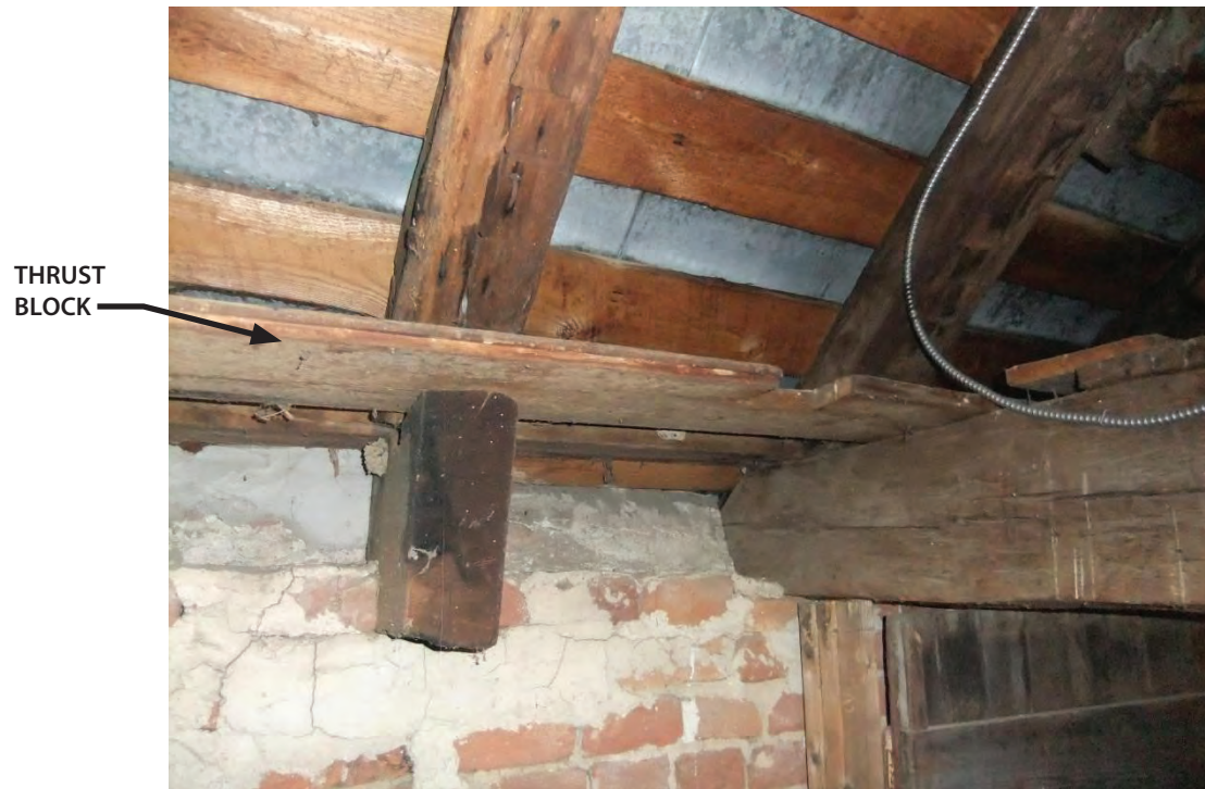
Figure 5: Roof rafter bearing at top of masonry wall. Note use of thrust block.
