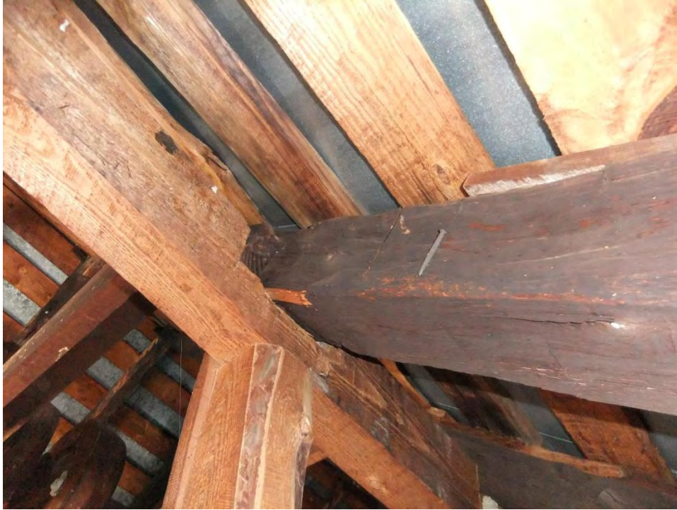
Figure 7: Purlin notch around existing rafter
