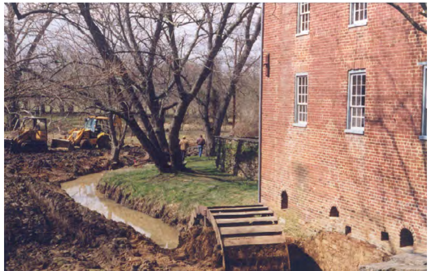
Waterford Mill, excavation of mill race, 1998 [WF].
