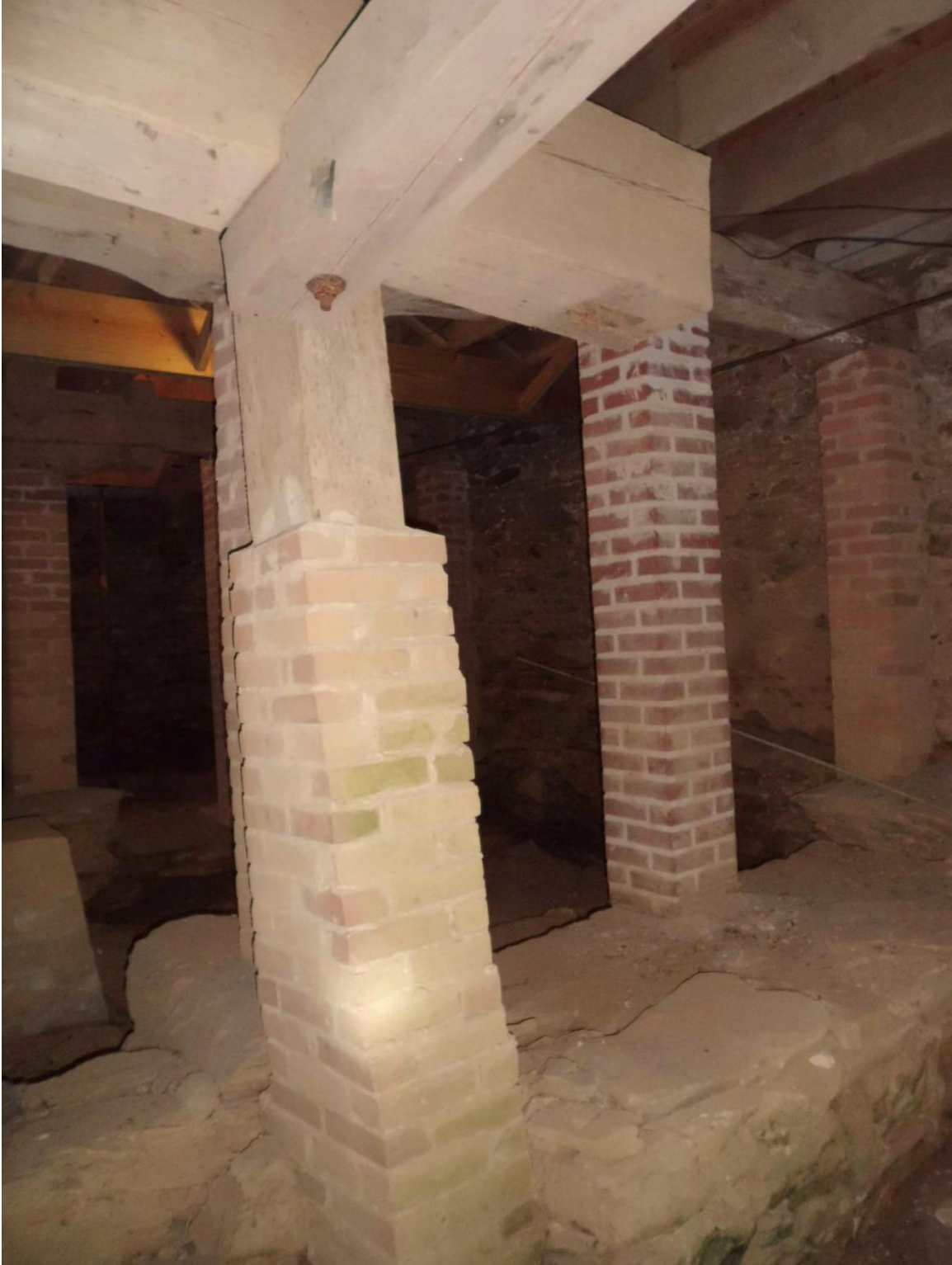
Figure 40: First floor canted brace masonry pier support
