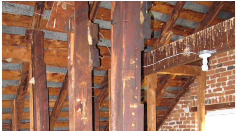
Grooves and notches in the vertical posts at the west end of the auxiliary drive shaft (located above) show where bevel gears connected to another drive shaft.
